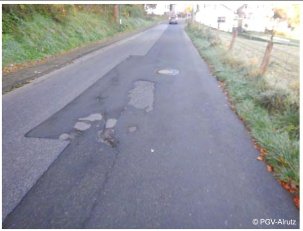
A photograph of a road surface showing significant damage and potholes, indicating the need for repair. The road is paved and has several large potholes and areas of missing asphalt. The damage is in the center of the road. The photo is taken from a low angle, looking down the road. © PGV-Alrutz                                            |
